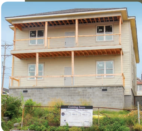
New Transitional Living apartment building under construction.
